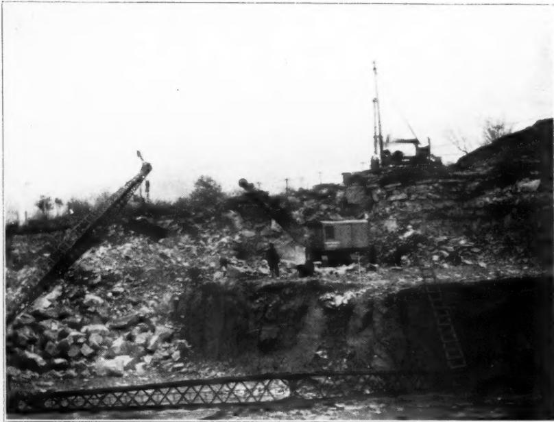
Northwest Shovel Stripping Overburden
